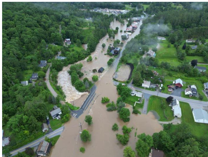
Flooding at Williams Dam with Overtopping Flow
