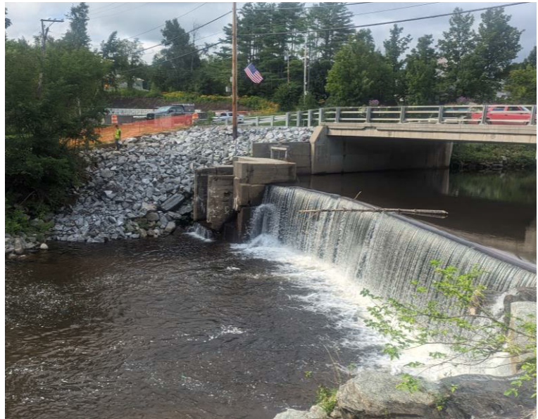
Repairs to Right Abutment/Route 11 Bridge Abutment
